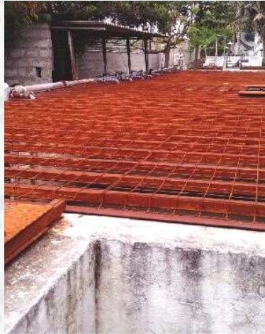
Sewage Treatment Plant
